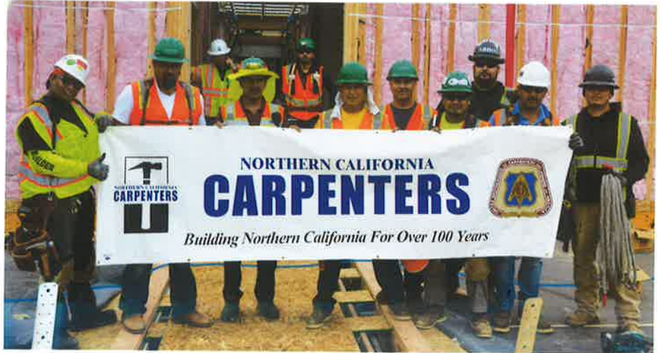
The Carpenter crew installing Factory_OS modules at The Union, working for Cannon Constructors, includes Evella Holt, Local 713; Dani Bugurin, Local 46; Gerardo Garcia, Local 217; Jose I. Garcia, Local 713; Edgar G. Romero, Local 713; Mauricio Poblano, Local 46; Jose Contreras, Local 22; Juan Carlos Hernandez, Local 46; and Laborers Joe Ramirez and Randy Ramirez.
