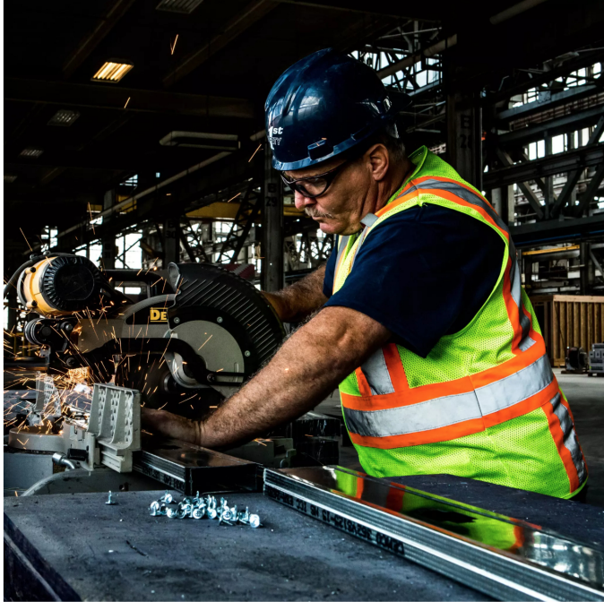
Jeff Anderton, a Factory OS worker, cuts ceiling framing that will be fitted into the modular housing units. Christie Hemm Klok for The New York Times
