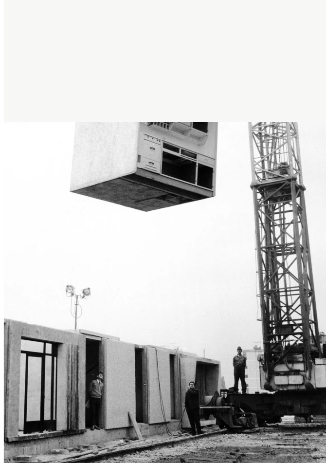
Prefabricated housing, in one form or another, has been around since at least the early 17th century, when Massachusetts settlers built homes of materials shipped from England. In the 1950s, Hungarian workers lowered a prefab kitchen at a housing construction site. Sovfoto/UiG, via Getty Images
