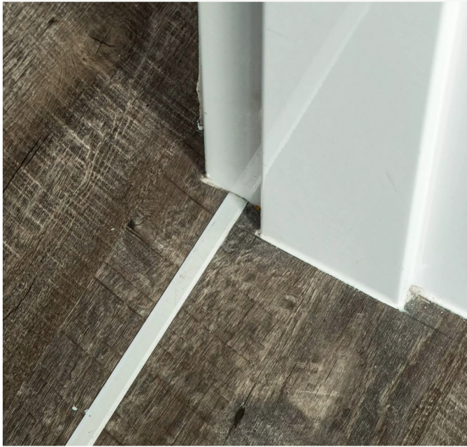
A telling detail that this is a prefabricated unit: the small strips in the door frames, designed to hide the connection between modules. Christie Hemm Klok for The New York Times
